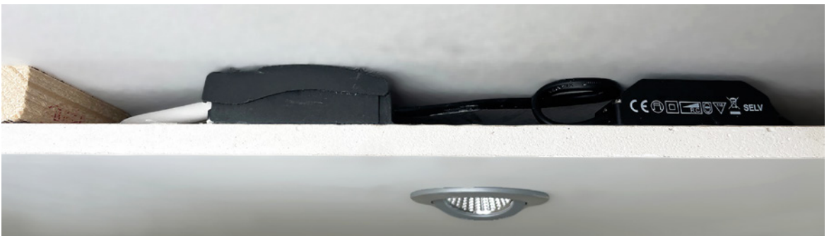
6 - The result: a compact installation with a swivelling spot, a dimmable power supply unit and the option of through-wiring in the ceiling cavity - ideal in refurbishment areas.
